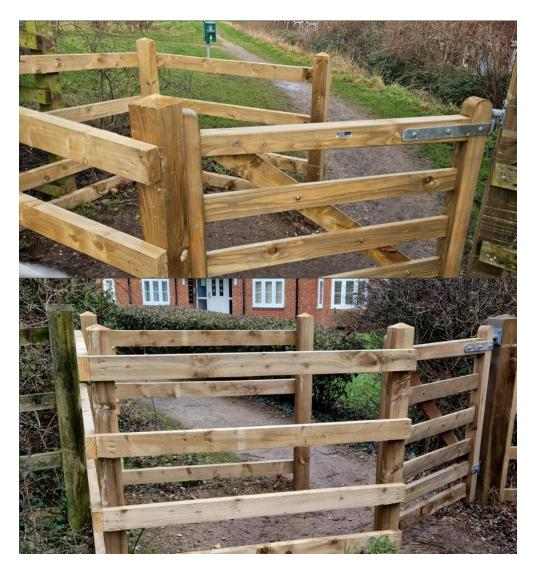
South Derbyshire District Council have recently updated the gates at either end of the Mease Meadow to both replace a rotten/broken unit at the Humber Street end and make both sets usable by wheelchair users and people with large pushchairs / strollers. They've been made wider and deeper to match ones elsewhere in the village. It's taken about 6 months from my initial
